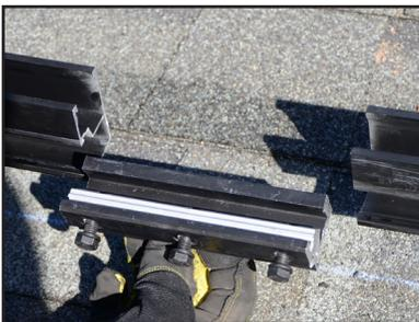
The rail splice is inserted into the channel where two rails but together. Three bolts are used to tighten the splice.
